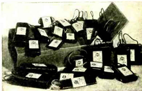
Fig. B This kit of filter and A.F. bypass replacement condensers meets any need of the Service Man; the units are in standard sizes and capacities.
