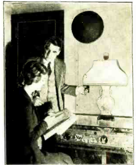
A typical room installation in the New Yorker Hotel. The wall plate under the man's hand contains the four-station selector switch and volume control; the reproducer cone is above it.
